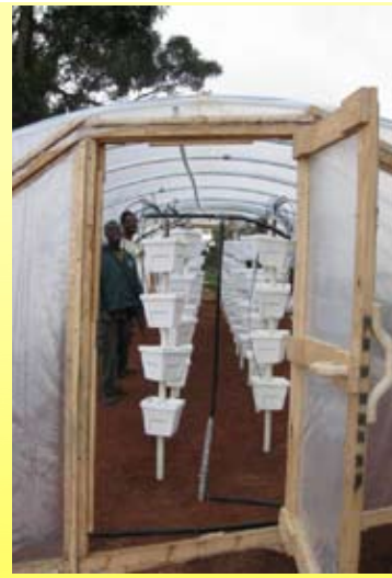
The completed hoop house is covered with plastic sheeting. It is shown here with the door open, revealing the vertical stacker system.
