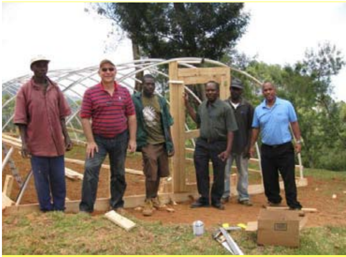
Brian Boman (second from left) and the Haitian Team pose before the hoop house under construction. Most of the materials for the hoop house had to be flown in from the United States, brought up the mountain in a truck, and carried the last few hundred feet of elevation. All photos on this page are courtesy of Brian Boman.
